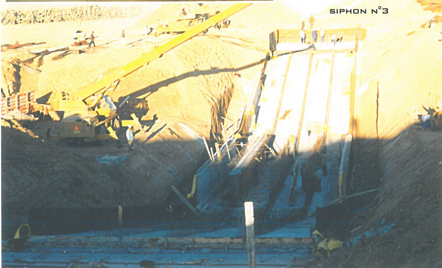
FERRAILLAGE RACCORDEMENT
